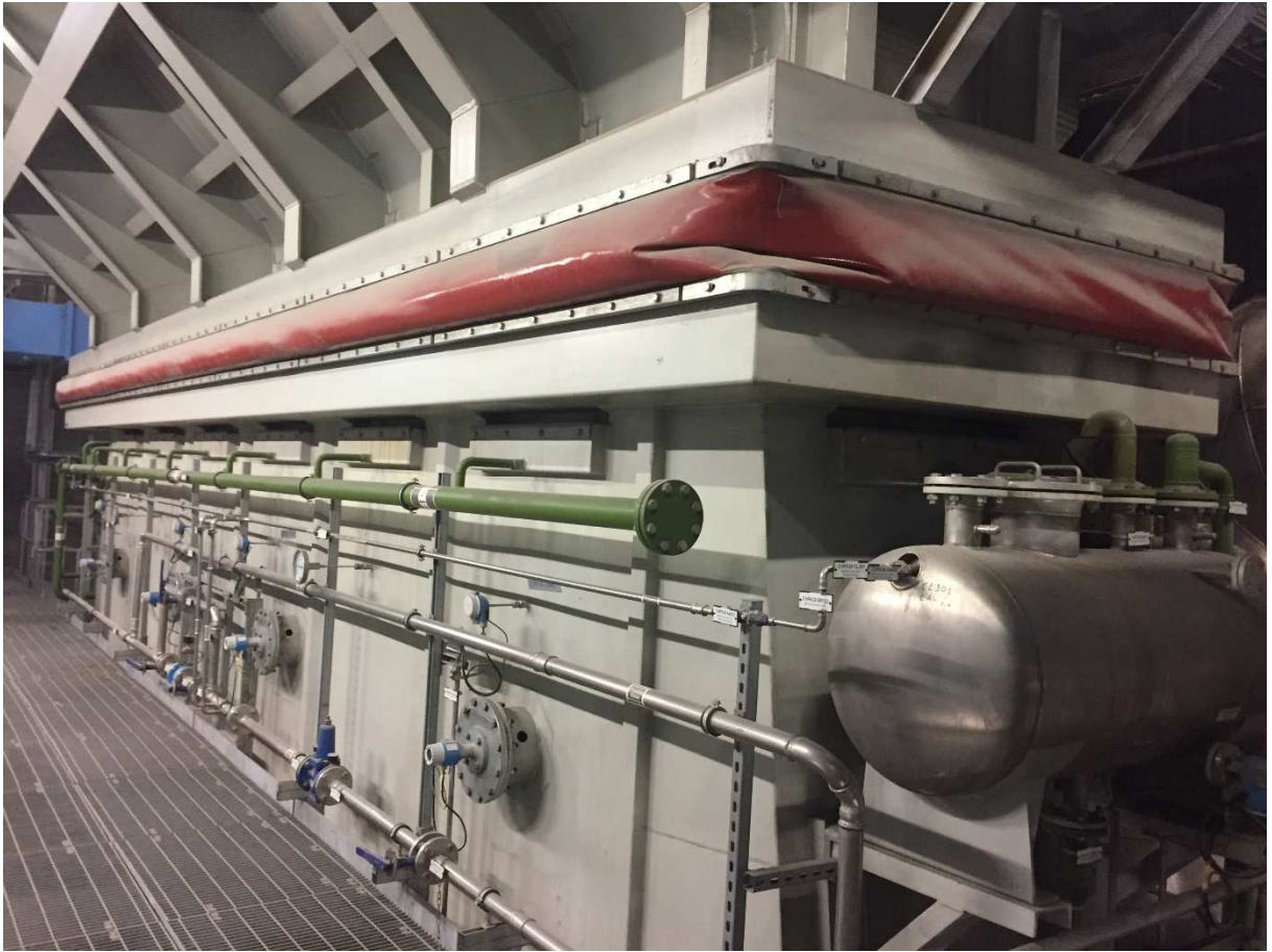
Plate 3.5: RRRF Waste Feeding Hopper
