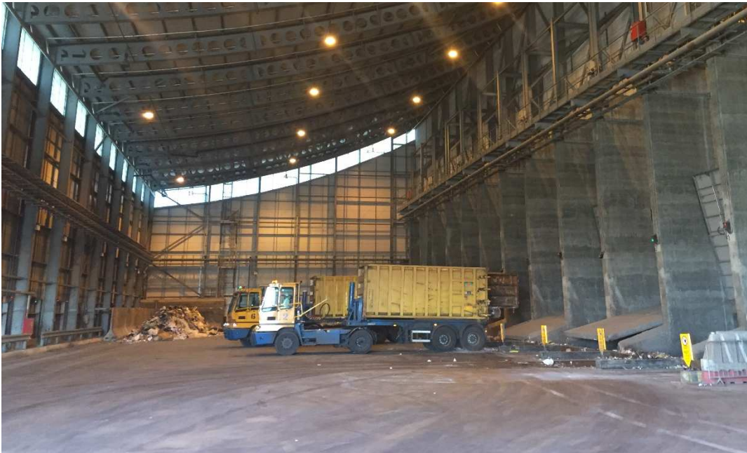
Plate 3.2: RRRF Waste Reception and Tipping Hall
