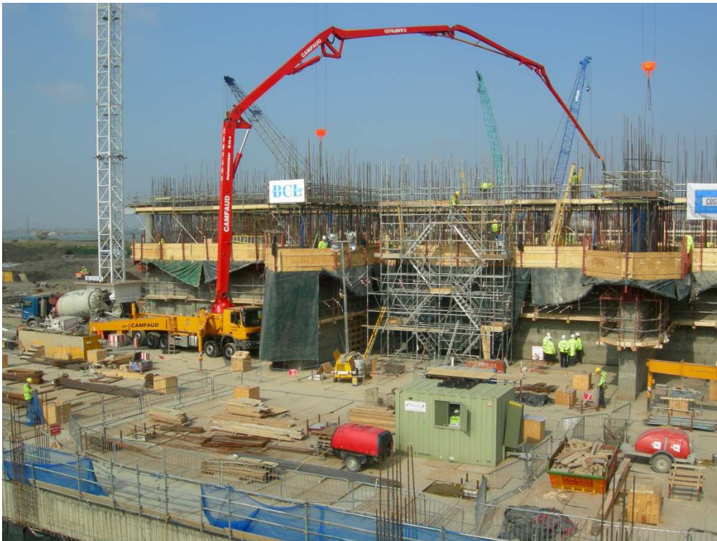
Plate 3.17: Typical bunker during a slip form operation
