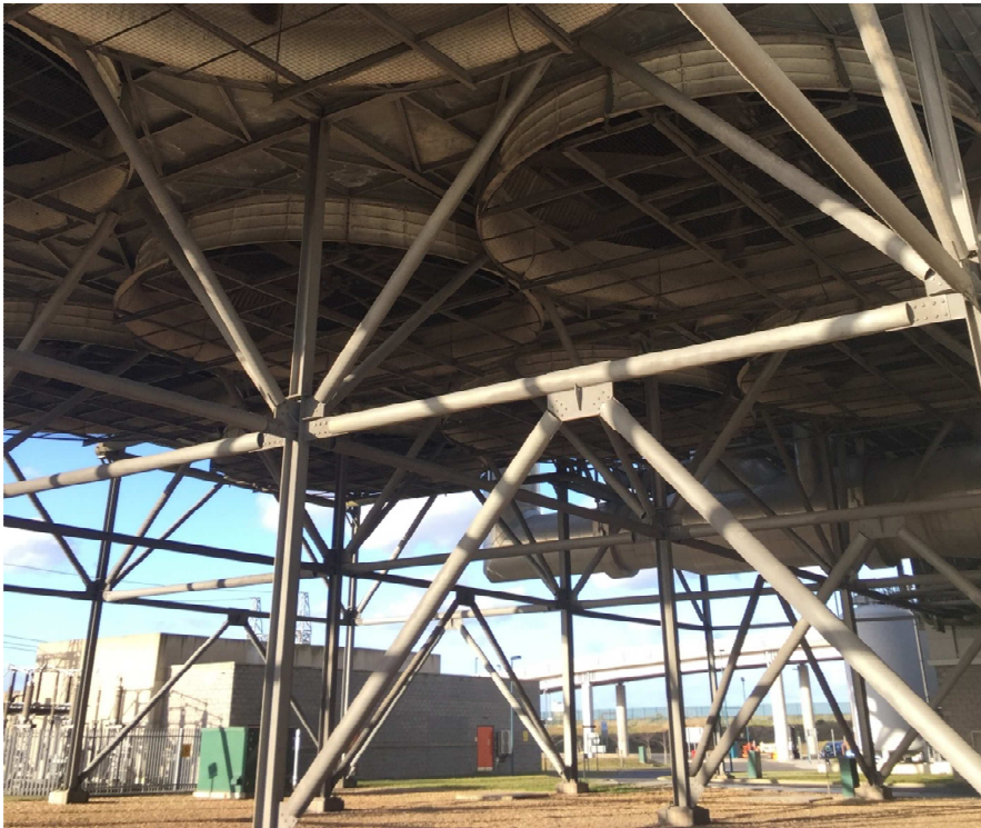
Plate: 3.10 RRRF Air Cooled Condensers
