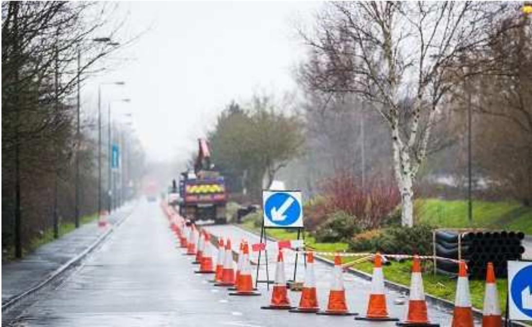
Plate 3.18: Example approach to cable working area
